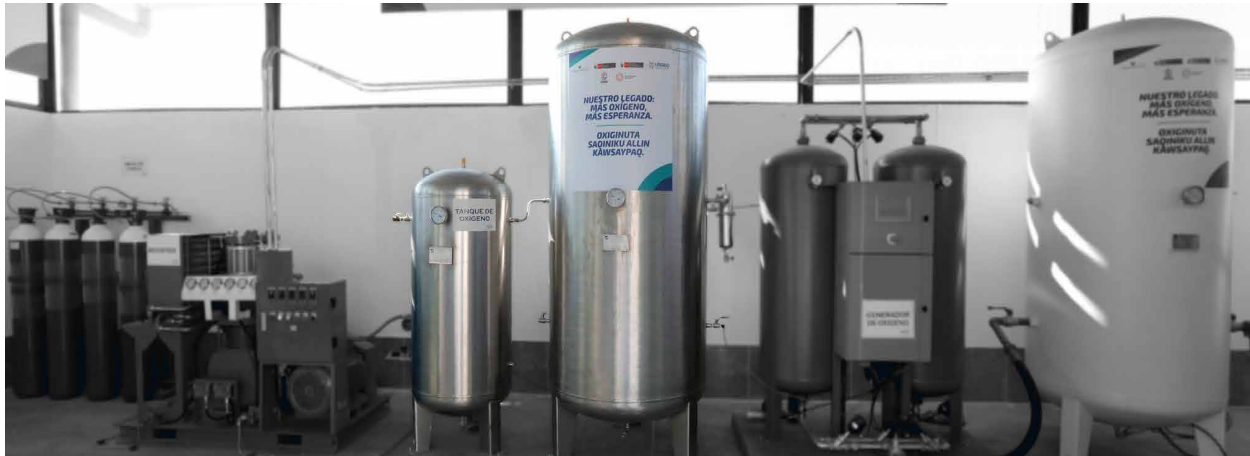
Figure 11. Tanks for oxygen storage produced by adsorption
