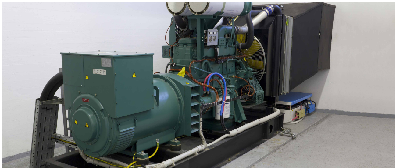
Figure 19. Emergency power generator
