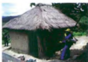
Techo material vegetal
