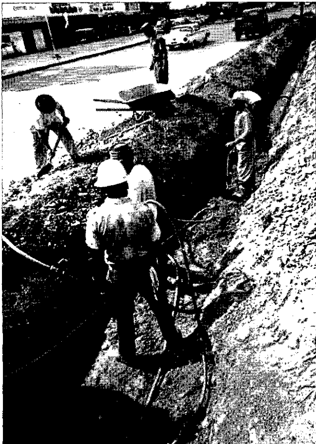
This pipe will carry water from Panamá City to the population of Río Abajo, Panamá.
