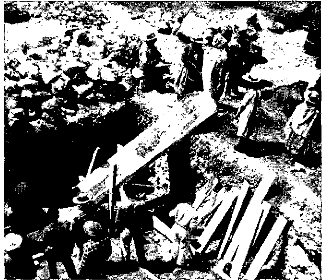
Paca, Junín, Perú: under the guidance of an expert, villagers build their own reservoir.
