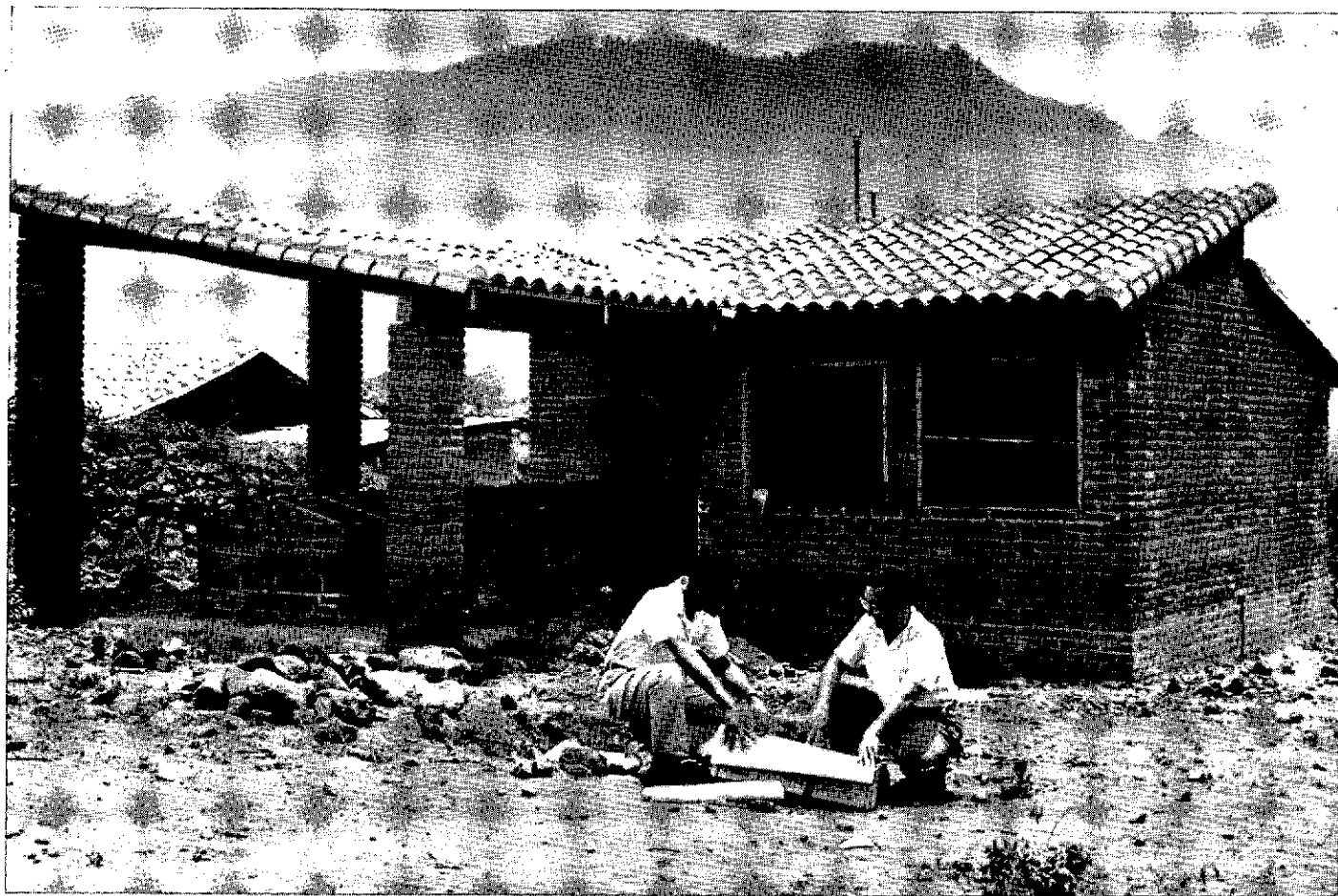
Constructing shower, latrine, and clothes-washing facilities for the people of a crowded suburban section of Tegucigalpa, Honduras. Work was done under the technical guidance of a PASB/WHO consultant engineer.
