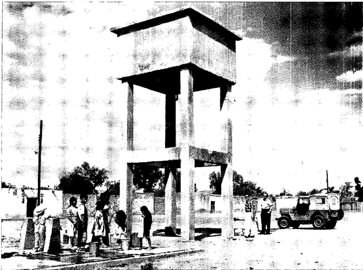
Water tank constructed by villagers under guidance of an engineer. The construction of some 400 similar tanks is planned over a four-year period in the State of Guanajuato, Mexico. Costs of operation and maintenance will be covered by monthly collections from householders. PASB/WHO assigned an engineer to this project.
