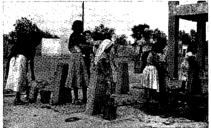
Six faucets to serve village residents. This basic water-supply unit will permit the residents to extend water lines to the rest of the village as rapidly as pipes can be obtained, Roque, Guanajuato, Mexico.
