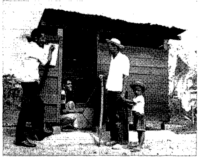
Two sanitary inspectors check post-construction maintenance of a rural latrine and shower combination, designed and constructed by sanitary engineers and personnel of the La Chorrera Rural Health Center, Panama.
