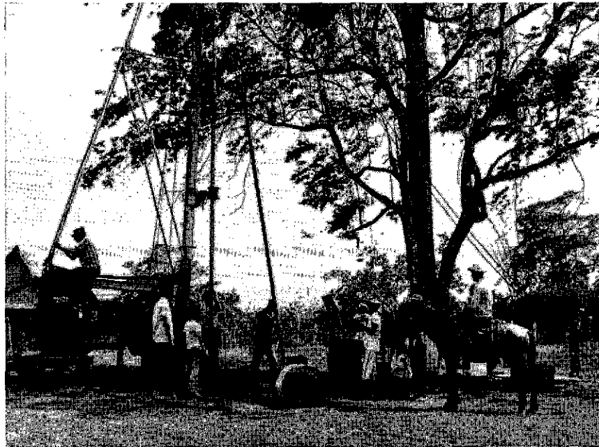
Approximately 265 inhabitants of this community will benefit from a new well being constructed under the supervision of the sanitary engineer of the La Chorrera Rural Health Center, Villa Rosario, Capira, Panama.
