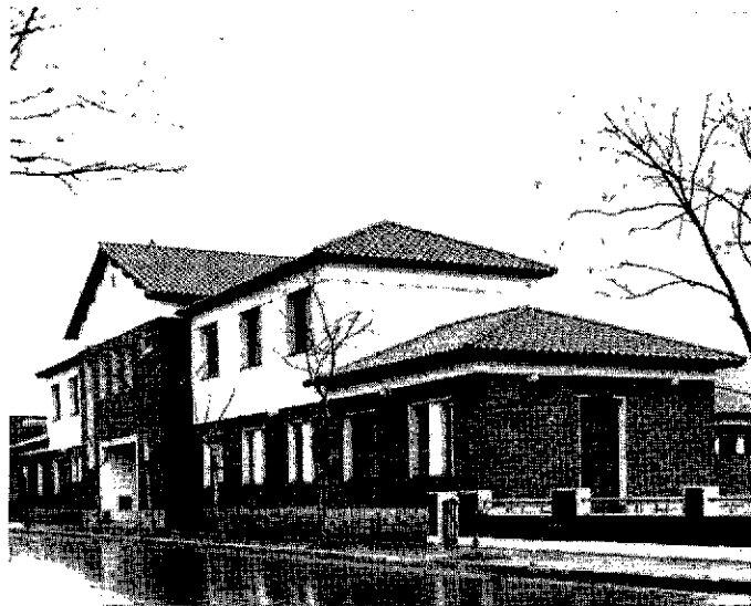
Main building of the Pan American Zoonoses Center, Azul, Buenos Aires, Argentina
