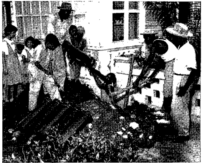
Installation of sewage pipes at a home in San Cristóbal—another project of the Health Center's Sanitation Section, San Cristóbal, Dominican Republic
