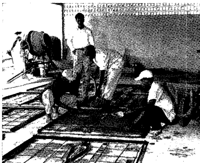
Chief of construction supervises the making of latrine platforms under a program of the Sanitation Section of the San Cristóbal Health Center, Dominican Republic
