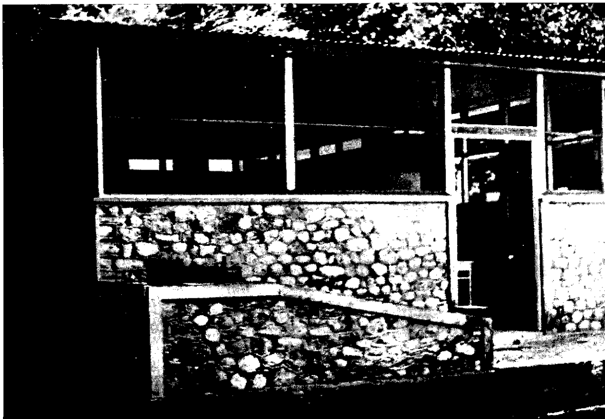
This modern dispensary was erected in place of the wooden shack which previously served as the clinic for the inhabitants of the Marbial Valley, Haiti
