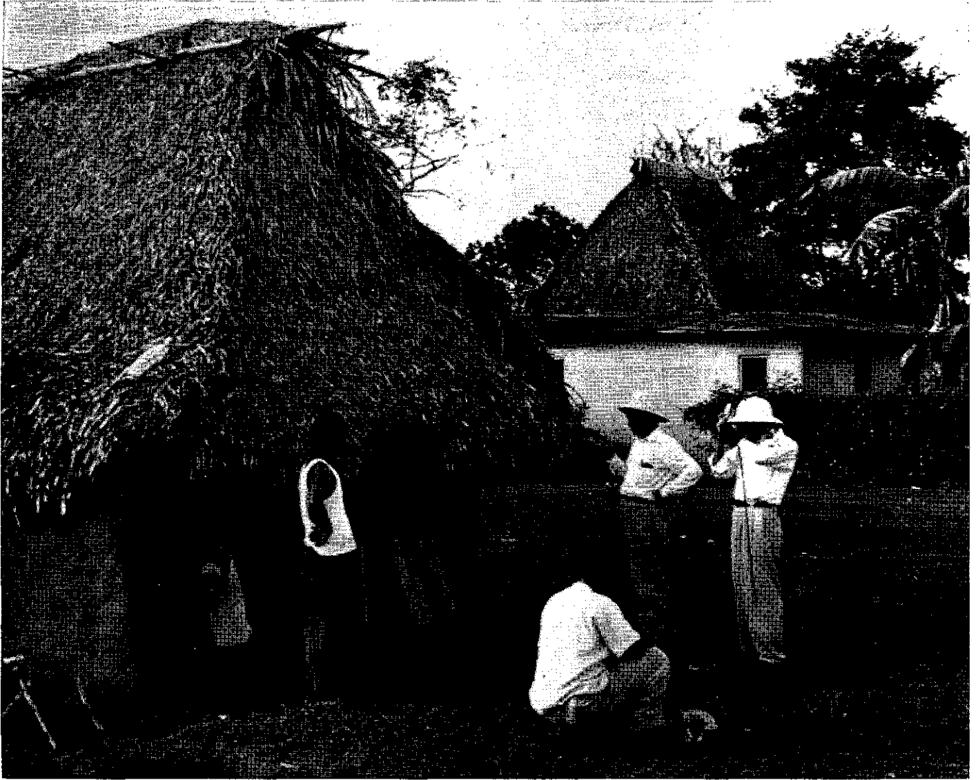
Streets being laid out by survey team, La Chorrera, Panama
