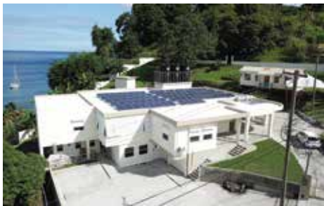
Completed modernization work at the Chateaubelair Hospital in Saint Vincent and the Grenadines, 19 February 2019.
