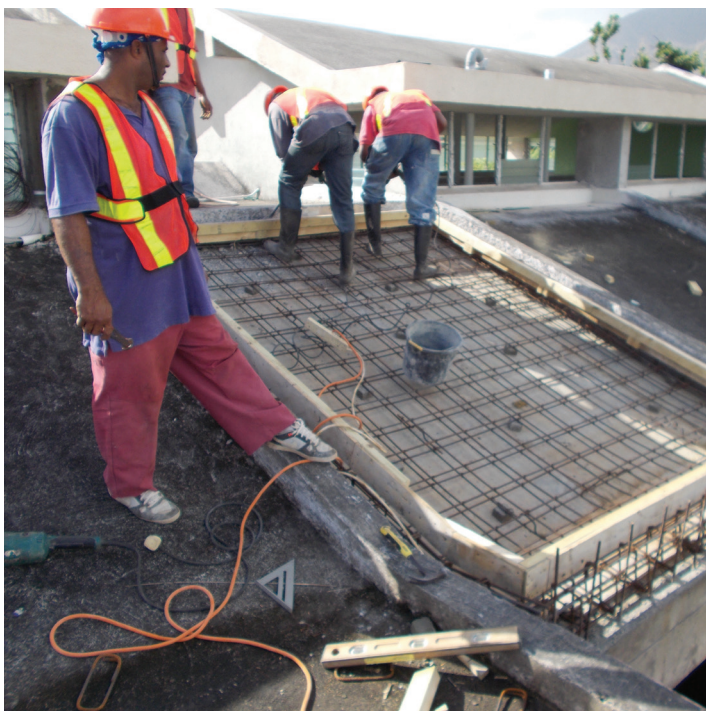
Installation of concrete ceiling in the La Plaine Clinic in Dominica
