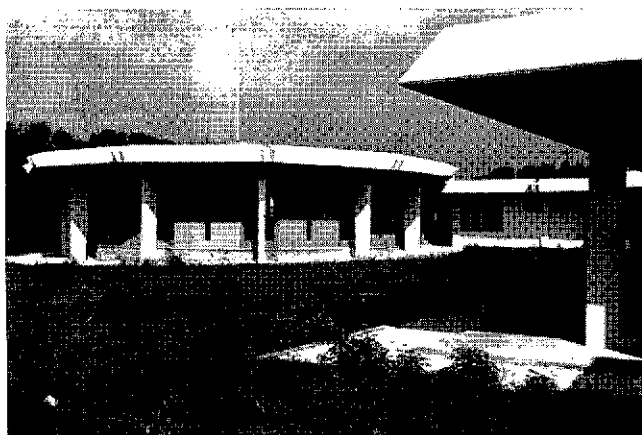
Building (under construction) for the School of Dental Nurses in Jamaica.
