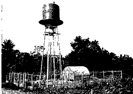
5. The tank and pumping station already installed.
