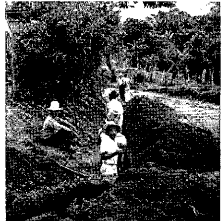
3. The trenches are dug with community help.
