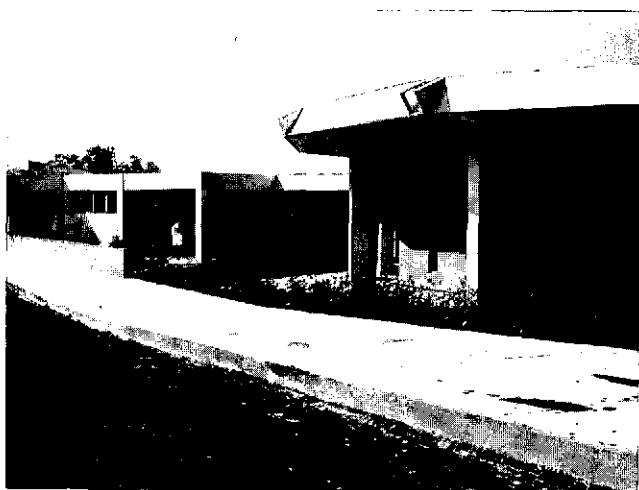
Building (under construction) of the School of Dental Nurses in Jamaica.
