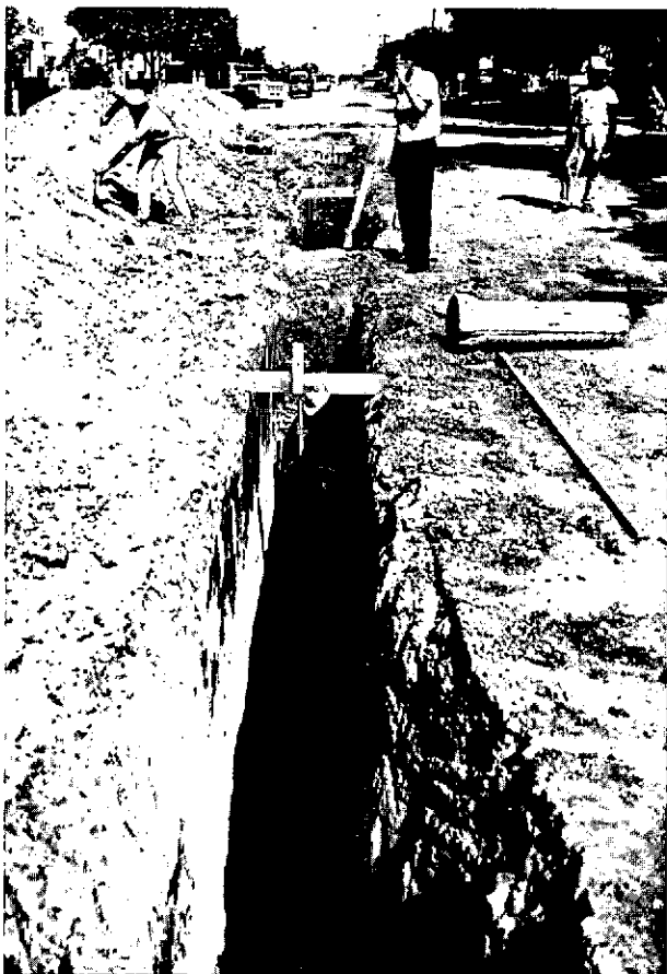
Digging of trench for installation of sewerage for a town of 10,000 inhabitants.
