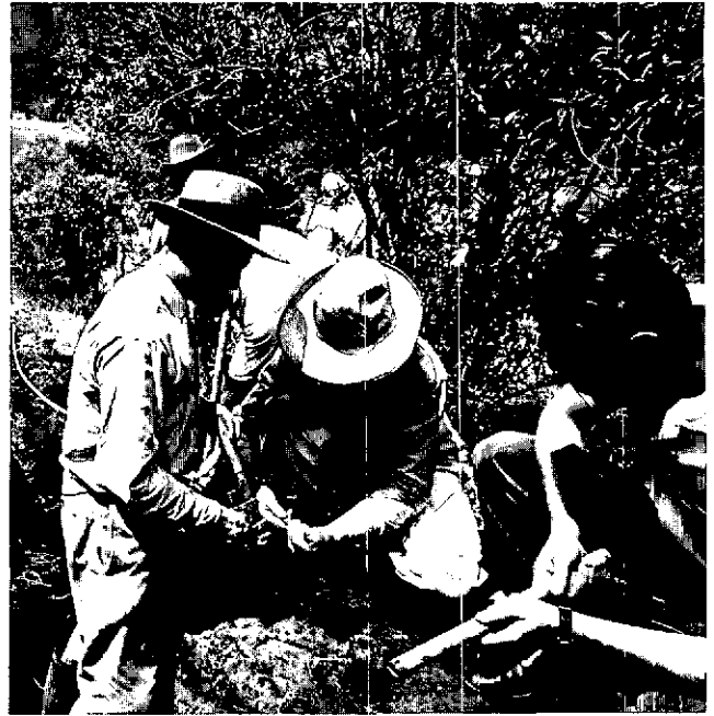
Village dwellers collaborate in the installation of polyethylene pipes for a community water supply system.
