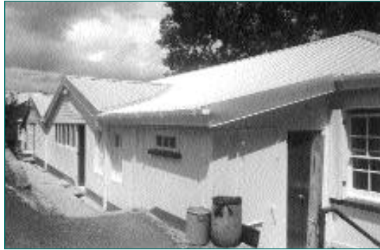
The Duncan Ward of the St. Georges Hospital, Grenada, retrofitted under the DIPECHO project.
