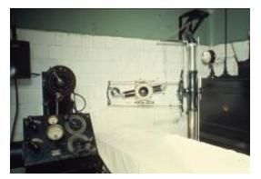
*Figure 3:* Argentina, 1965—Inadequate filtration and excessive tube housing leakage.
