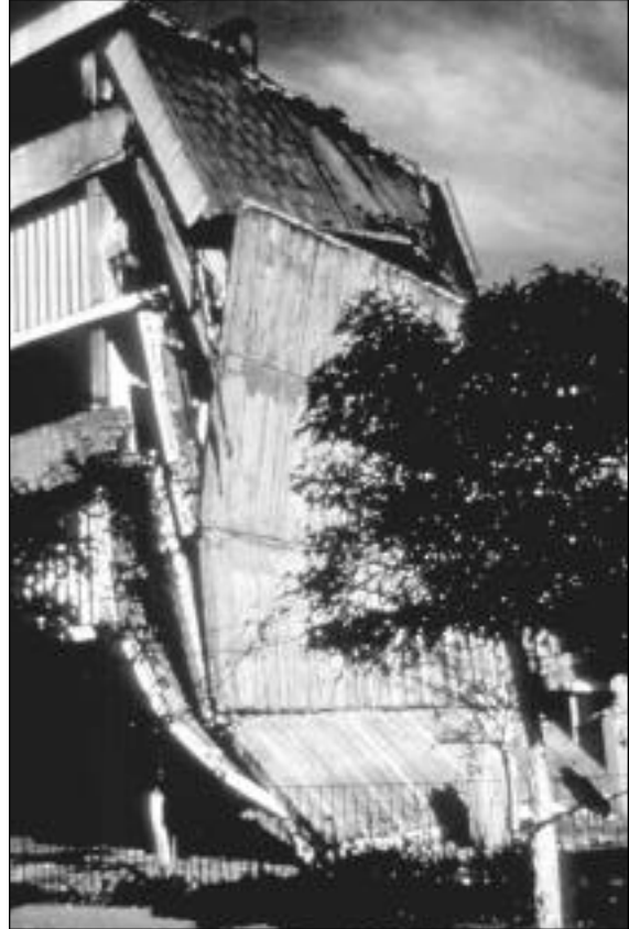
Photograph 11. Structural collapse due to the discontinuity of vertical elements.
