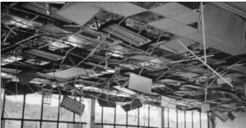
Photograph 19. Damage to ceilings
