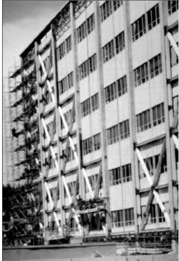
Photograph 13. Reinforcement with diagonals.
