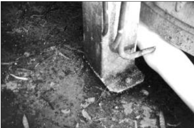
Photograph 16. Detail of support connections for liquid oxygen tank.
