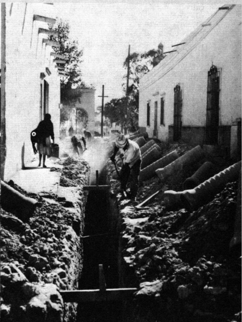
Top: Child drinking from pump in a rural village. Bottom left: Laying pipe for a water supply system. Bottom right: Excavation of ditches for sewerage.
